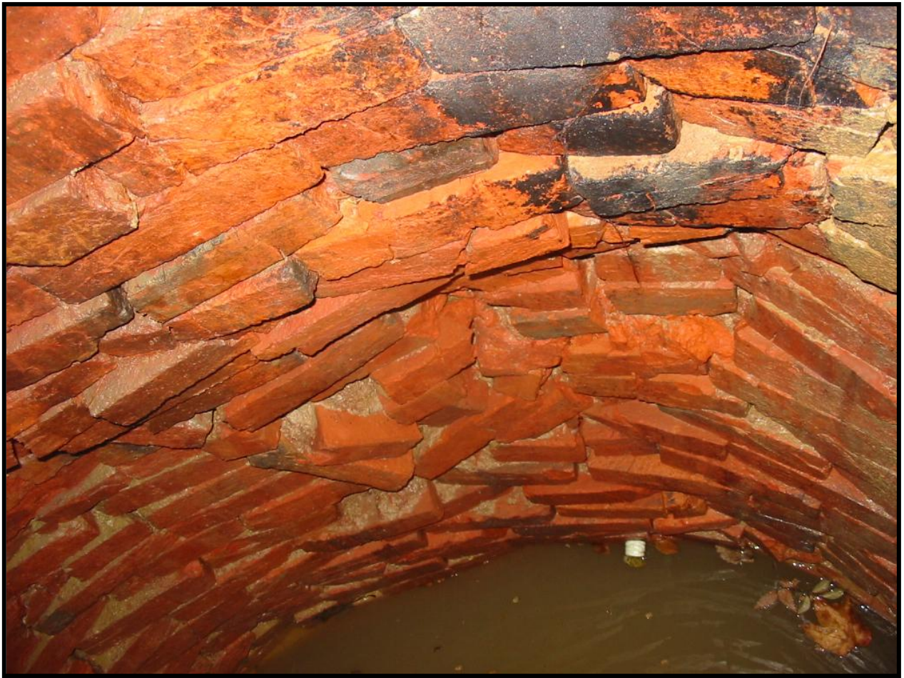
Photographic Plate 5: Interior of Feature 29, the Dut , showing collapsed brick. Photo facing north, 24 November 2008.
